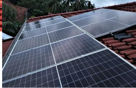
Panel Installation Jinko Mono Half Cell Module -20 Nos
