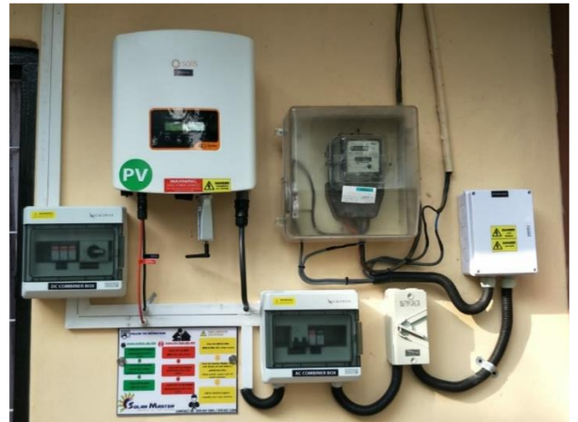
Inverter Installation Solis Single Phase 3kW
