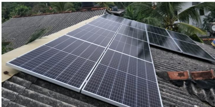
Panel Installation Jinko Mono Half Cell Module -12 Nos
