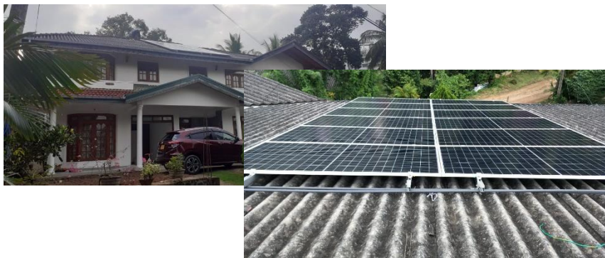
Panel Installation Jinko Mono Half Cell Module -12 Nos
