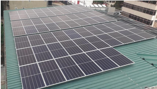
Panel Installation Jinko Mono Half Cell Module -89 Nos
