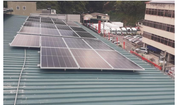
Panel Installation Jinko Mono Half Cell Module -89 Nos
