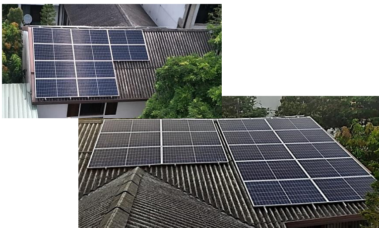
Panel Installation REC Mono Cell Module -26 Nos
