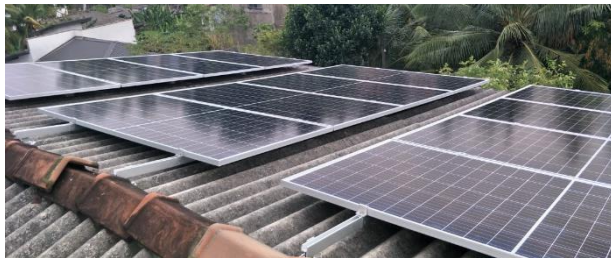
Panel Installation REC Mono Cell Module -12 Nos
