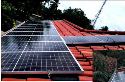
Panel Installation Jinko Mono Half Cell Module -20 Nos
