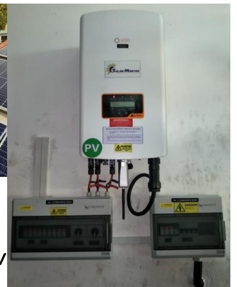
Inverter Installation Solis Single Phase 3kW
