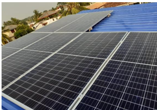
Panel Installation Jinko Mono Half Cell Module -06 Nos
