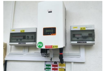
Inverter Installation Solis Three Phase 20kW
