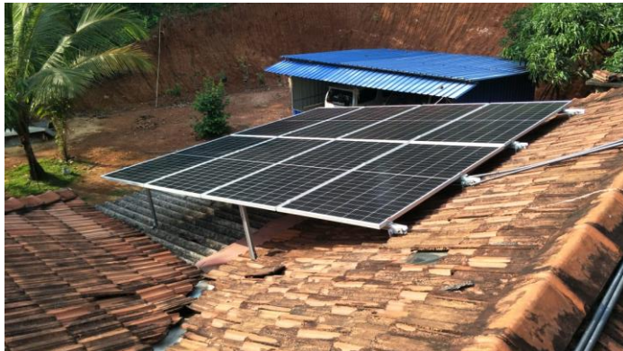
Panel Installation REC Mono Cell Module -8 Nos
