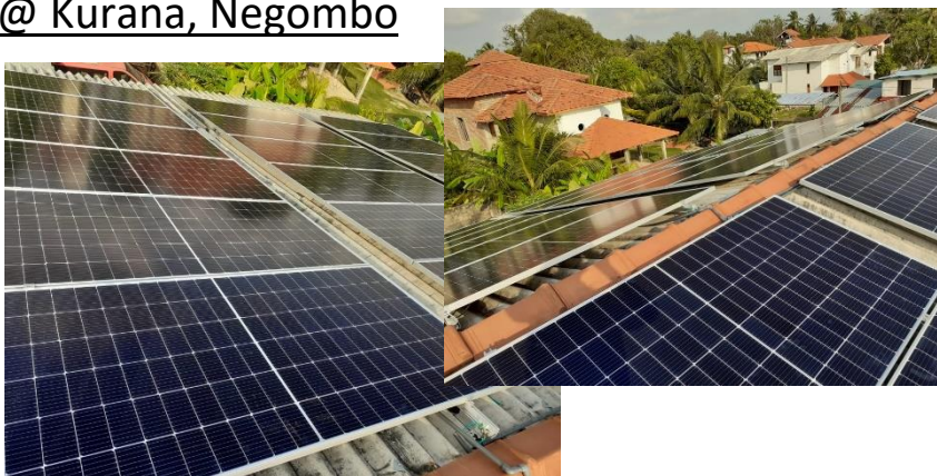
Panel Installation Jinko Mono Half Cell Module -30 Nos
