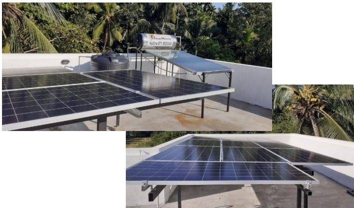
Panel Installation Yingli Poly Crystalline Module - 10 Nos
