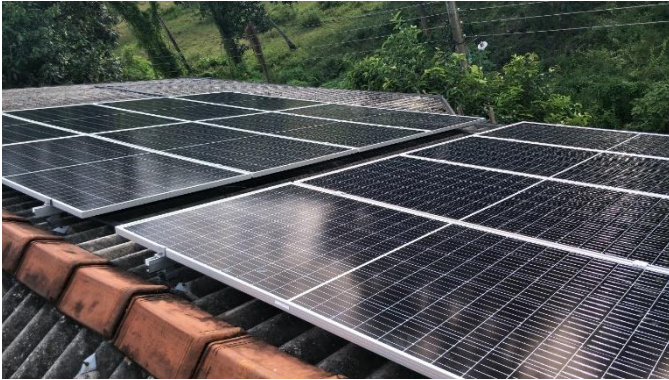
Panel Installation Jinko Mono Half Cell Module -12 Nos
